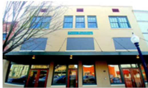
Figure 5.11d: Lofts in Downtown Bryan. Source: https://www.perrypropertiesinc.com/
