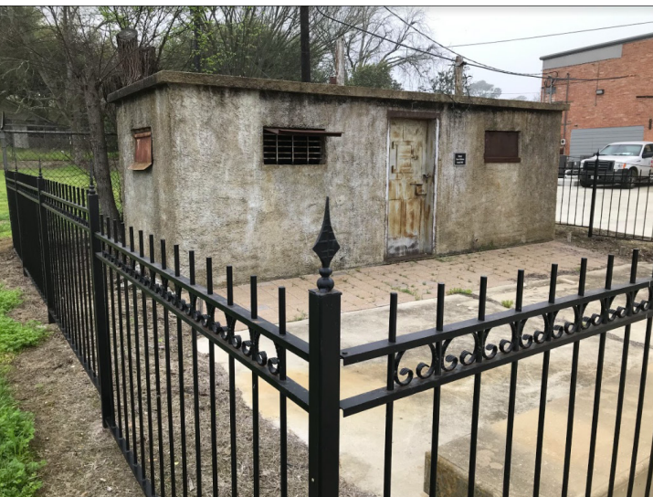
Figure 8.14 Calaboose Photo courtesy of the City of Caldwell
