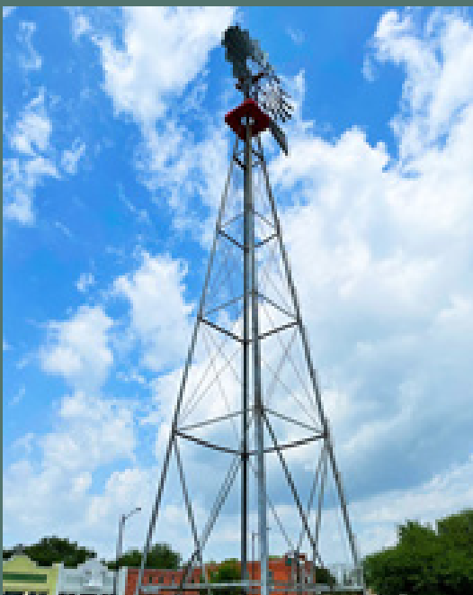
Figure #.# Old Garison Windmill restoration, Buda, TX Source: https://smcorridornews.com/buda-restores-and-relocates-old-garison-windmill/
